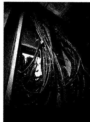
NETWORK CABLE: about 10 miles' worth in total.
