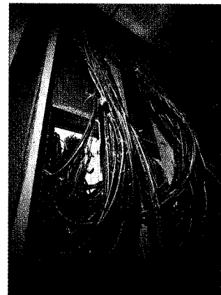
NETWORK CABLE: about 10 miles' worth in total.
