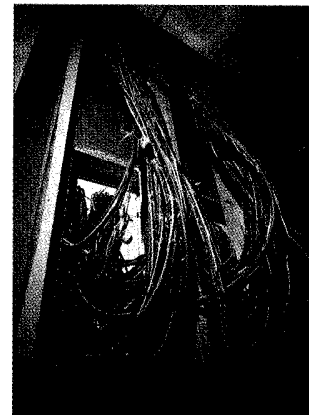
NETWORK CABLE: about 10 miles' worth in total.
