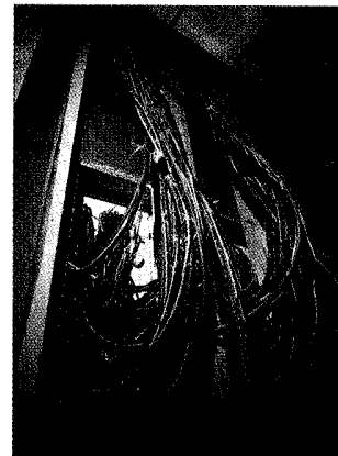
NETWORK CABLE: about 10 miles' worth in total.
