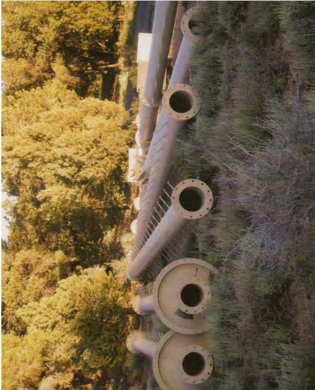
Figure 6: The proposed monopole structures have a tapered design with a base diameter of twenty (20) inches and a tip diameter of ten (10) inches. Final design, as recommended by staff, will be pursuant the approval of the building department.
